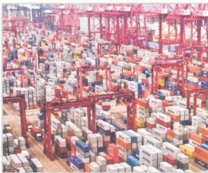
Hong Kong International Terminals
